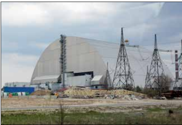
The Chernobyl power plant. Photo: Sylvester Nagorka.
